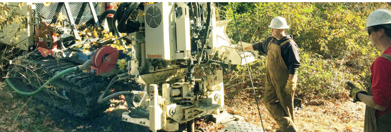
Test well being drilled at Cammett Way (USGS)
