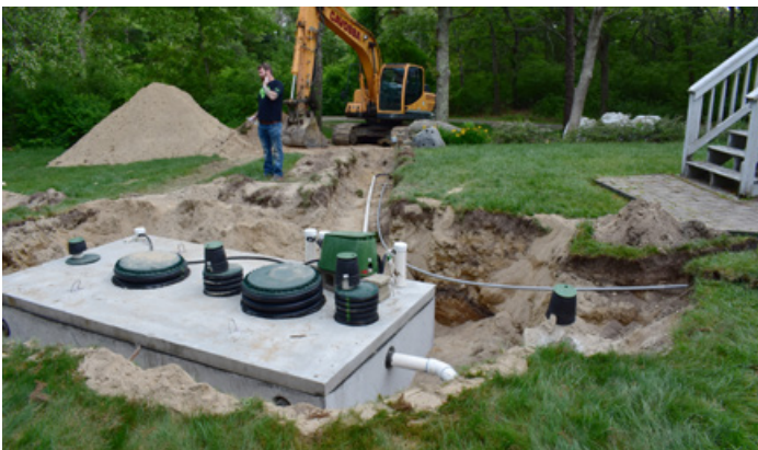
Before and after photos of a NitROE WWTS installation.
