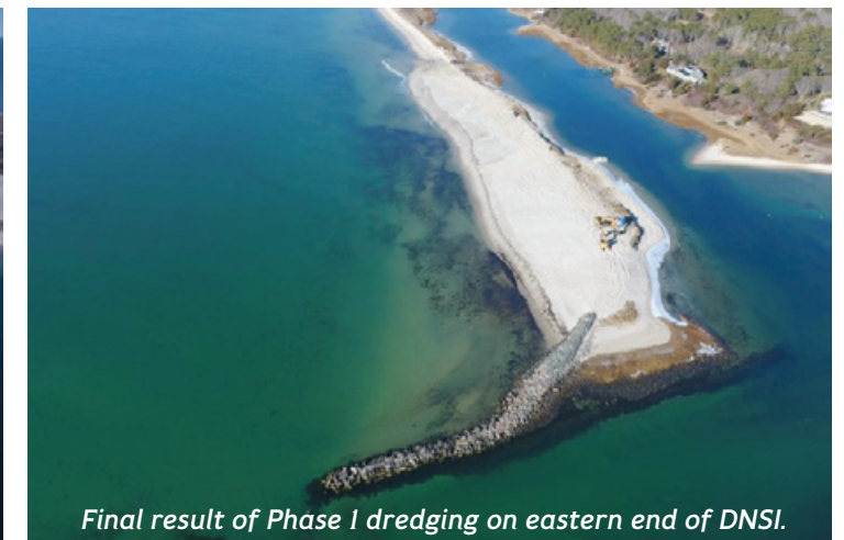
Final result of Phase 1 dredging on western end of DNSI
