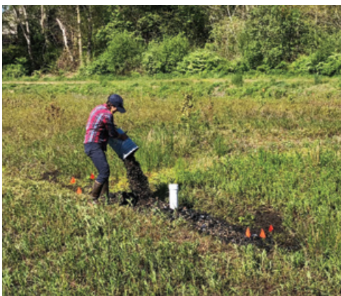
(Left to Right) Special Projects Manager Casey D. Chatelain prepares bog ditches in advance of the biochar bioreactor installation. BCWC Volunteer Tess Prete and Field Operations Manager Meg Materne fill wheelbarrows with the biochar/woodchip mix. Rachel Rubin, post-doctoral researcher from Mount Holyoke College, pours the biochar/woodchip mix into the bioreactor. BCWC volunteers Tess Prete and John Thomas work with Rachel Rubin constructing one of the three new bioreactors. After a long day's work, the first bioreactor is complete and already filtering water flowing through the bogs.
