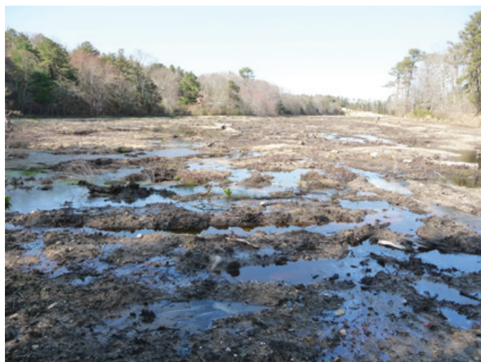
The site graded after sand was removed, ditches were filled, and sediment was moved (2010).
